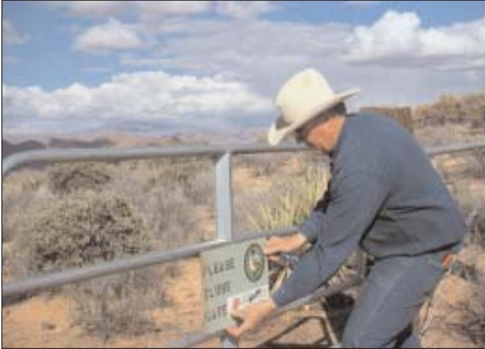
Arizona Trail Association Board Member, Terry Horne installs gates in Pinal County. Photo by Larry Snead, Chief Trail Steward
